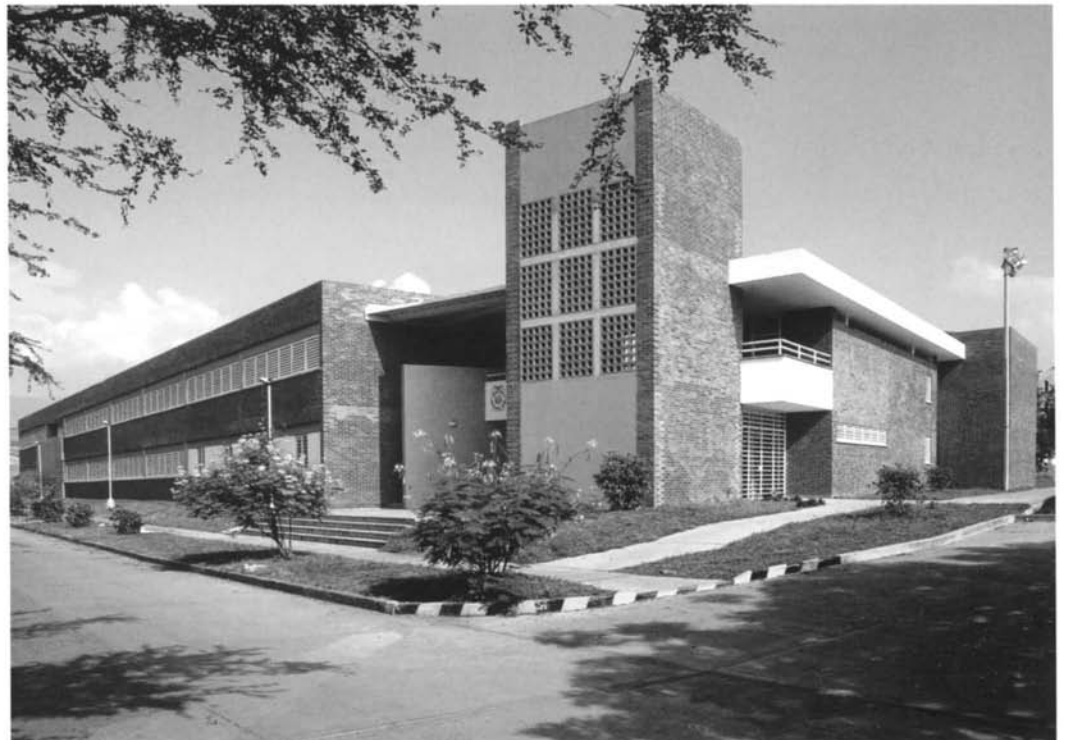
The colonnade provides shade for the classrooms | Entrance corner with stair tower for cooling and ventilation | Views of internal courtyard showing restrained use of colour
