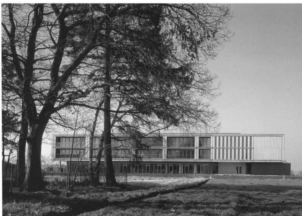
View towards the main entrance | Elevation from the riverbank | View to internal courtyard with broad steps running up to first floor teaching areas | View of typical classroom, with the use of simple materials and even controlled colour coding
