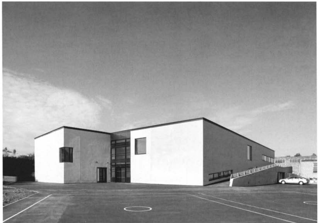
The school building is located on a steep embankment | Main entrance elevation with access ramp | Views of top-lit central circulation spine
