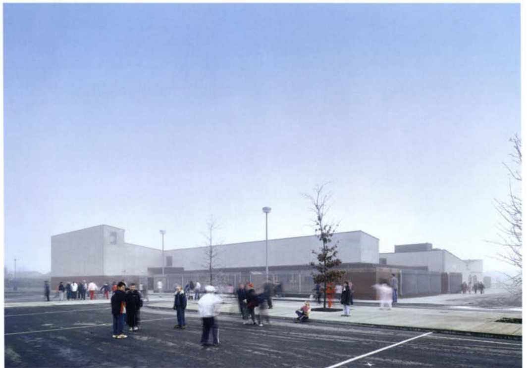
External view of the classroom 'dens' with their own gardens | View looking towards main entrance with perimeter security fencing integrated into the architecture | Vision panels in corridors | Internal view showing classroom work area with rooflight | Multi-purpose hall
