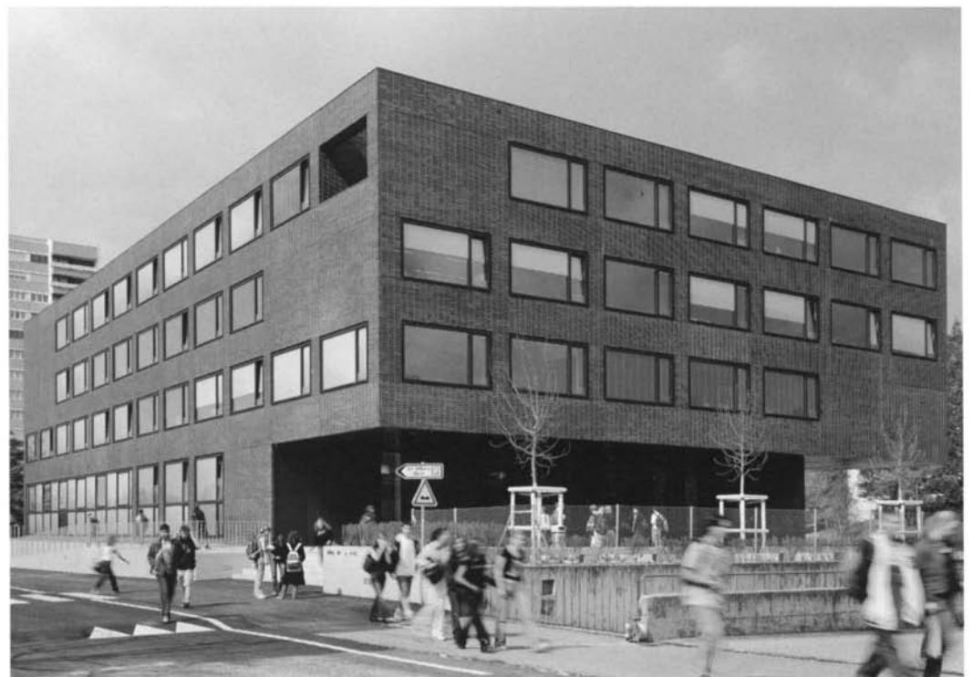
Cantilever with entrance beneath | View of entrance and street elevation | Views of the building from the northeast
