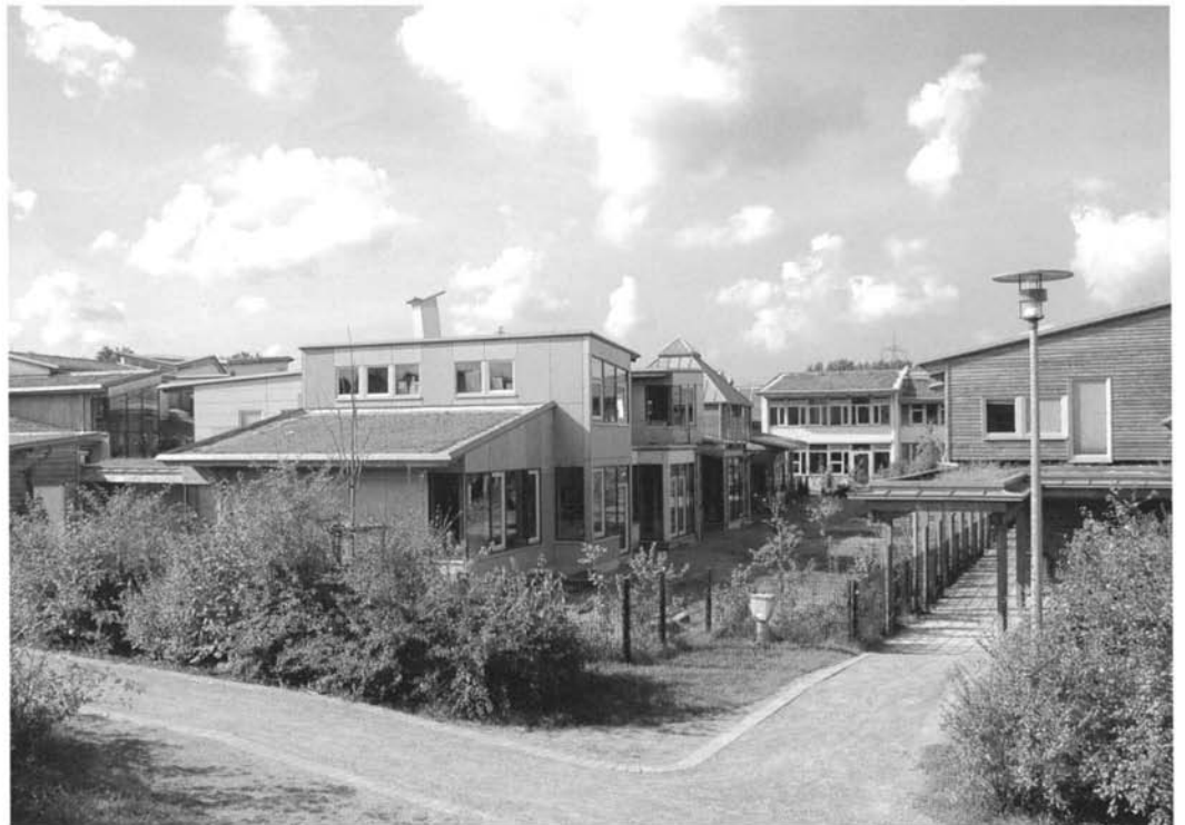
Linked classroom pavilions looking onto the meadow gardens | Classroom blocks combine to a rich variegated architecture which looks nothing like a conventional school | Exterior views
